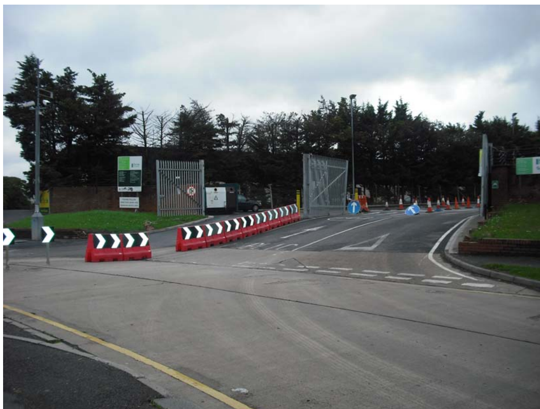
Waste site entrance
